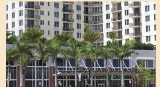
The elevated amenity deck ensures privacy for residents.
