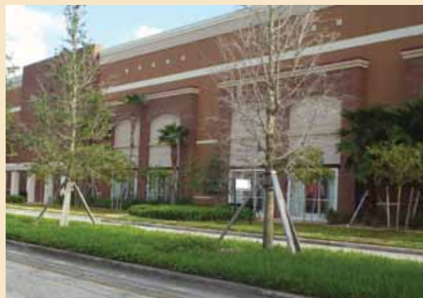
Façade treatment on rear of Kohl's store (north elevation).
