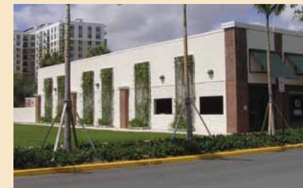
Temporary façade to maintain aesthetics between phases.
