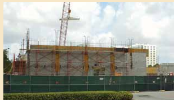
New buildings under construction.
