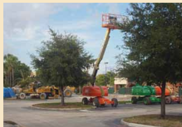
Future linear park used for staging area.
