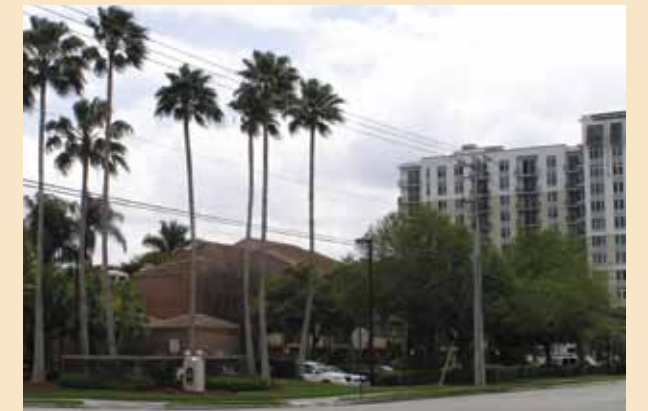
An easement for crane swing over the adjacent hotel was required to construct the high-rise residential building.
